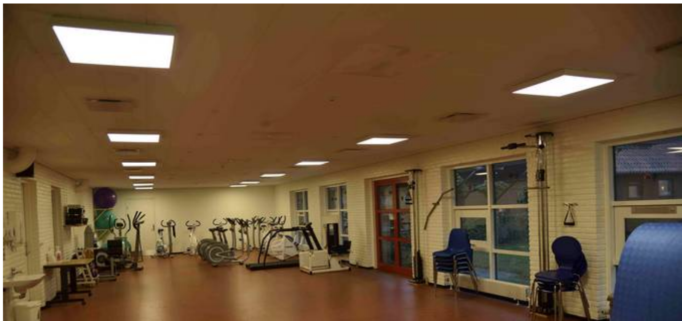
600x600mm paneler monteret i kassetter
